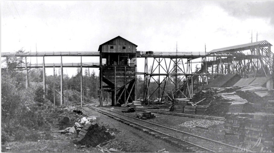
Mine B's storage bunkers were built above the train tracks. Judging by the amount of lumber in the foreground, this photo was likely taken while under construction.
