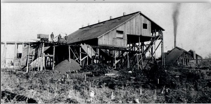
Mine No. 2's bunkers circa 1890. Mine #14 is to the right in the background.
