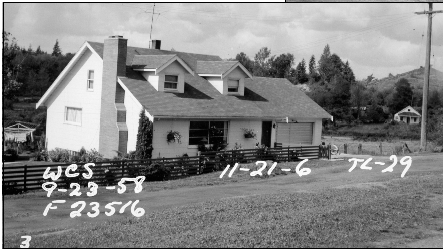
“Kuzaro” Home, September 23, 1958. King County Assessor photo of tax parcel number 112106-9029.
