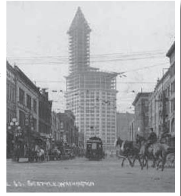
The Smith Tower under construction 1913.
