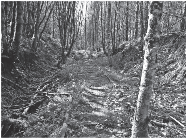
"Rusty Rails" (segment of abandoned rail line), Black Diamond, April 2018 photo by Robert Dobson
