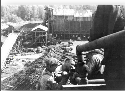
Archie Eltz, Charlie Falk, and Frank Merritt atop the rock dump working on a water pipeline, August 1949
