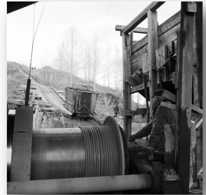
Frank Manowski to the right as the coal car climbs the slag pile, Jan. 1973.
