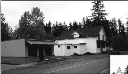
RedLine Mechanical next to Mama Passerilli's that's being remodeled
