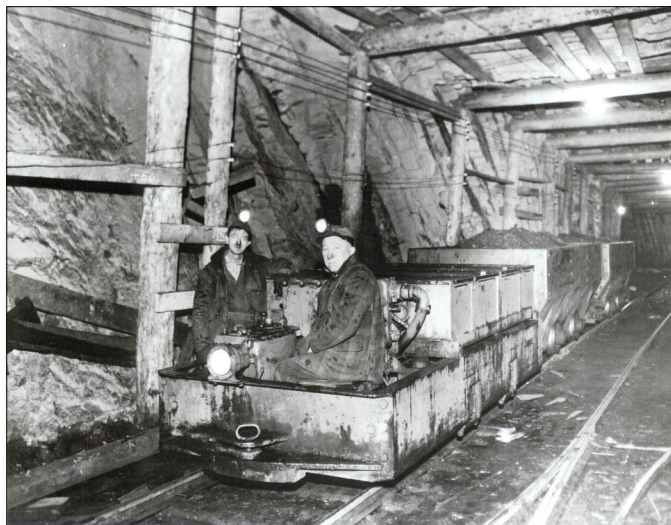
An electric motor pulls loaded coal cars through the gangway of the Wilkeson mine, March 18, 1944. Photo #D17170-21 courtesy of Tacoma Library.
