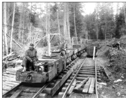
An electric motor hauls a train of coal cars to the plant near Ravensdale Lake. Photo #53911 courtesy of the Washington State Historical Society, Tacoma.
