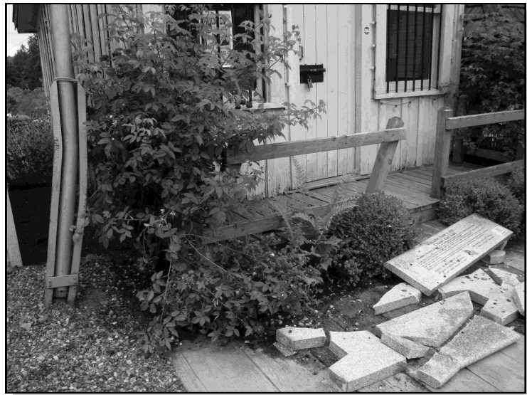
Damage to the granite benches, flag pole and jail from an early morning auto accident.
