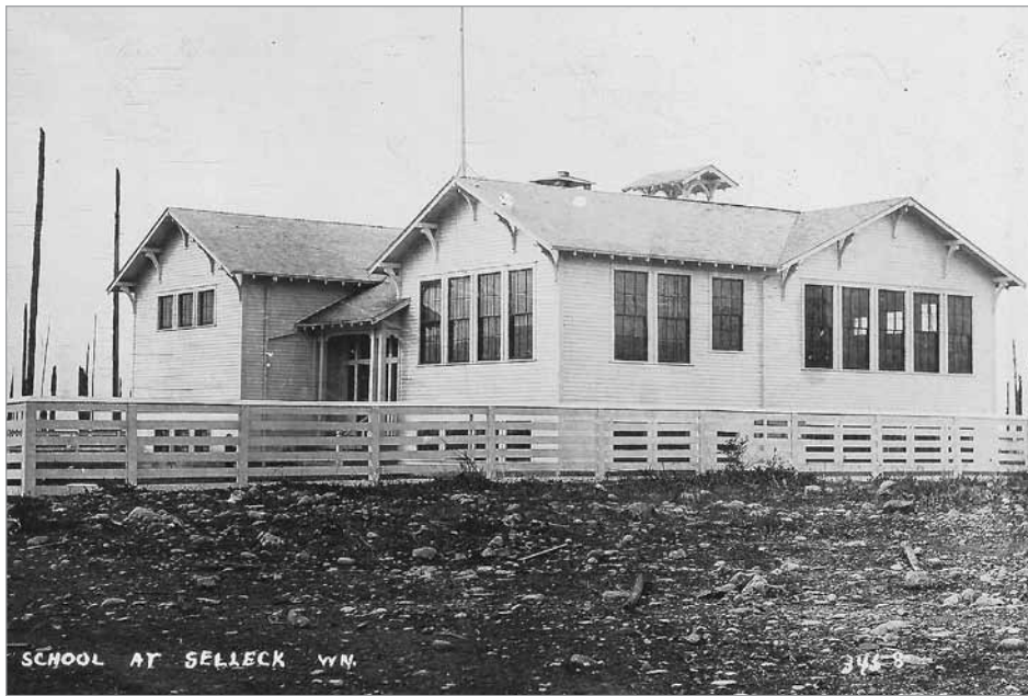
This school was destroyed by fire on December 31, 1929. (Photo courtesy of Art Van Bergeyk.) The “new” Selleck School was built in 1930 on the same site.
