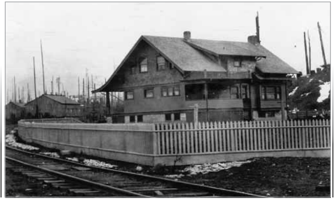
Frank Selleck's residence, also known as the superintendent's home. This Craftsman house features a full-length covered porch and a large shed dormer on this slope of the broad gable roof. (Photo courtesy of John Cooper.)
