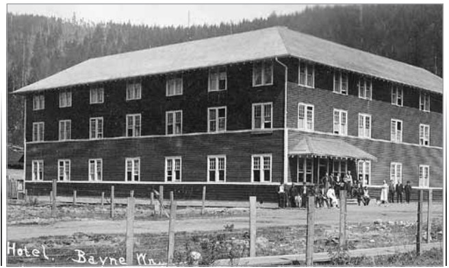
The three-story hotel had well constructed rooms, reading room, lobby, and dining room. Adjoining the hotel was a small two-story annex in which the help lived. The hotel accommodated 175 men.
