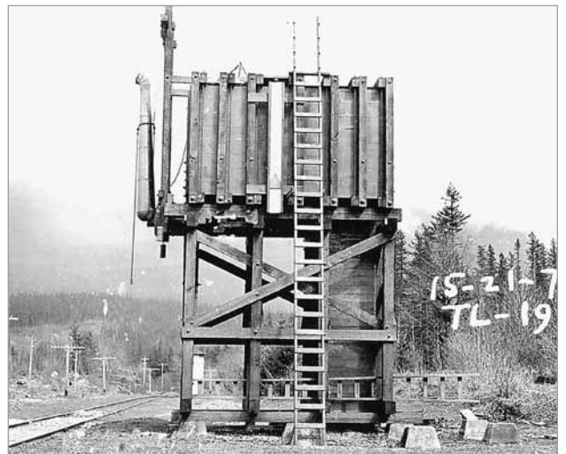
Shown here is a typical water tank for filling the tanks of steam locomotives, located along the tracks of the Northern Pacific Railroad between Palmer and Bayne. This April 1940 photo of King County Assessor tax parcel #152106-9019 comes from the Puget Sound Regional Archives.
