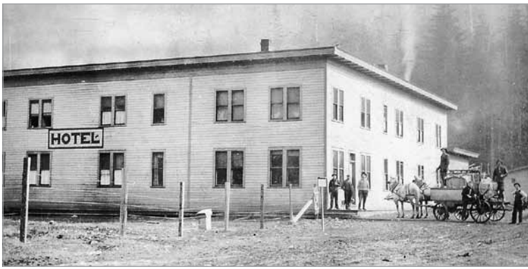
The hotel, which was operated for the accommodations of miners employed in the Carbon and Daly mines, was originally a two-story structure, but a growing work force necessitated an expansion.
