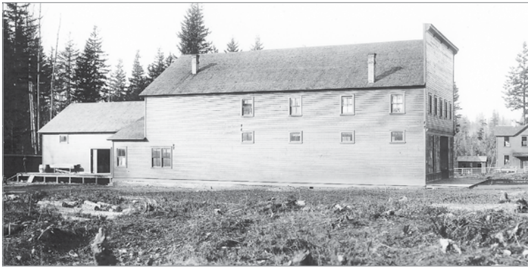
The company store building was originally located on Lawson Hill on a railroad spur that served the Lawson Mine. The store was moved to Railroad Avenue around 1911 or 1912 using horses and a windlass.
