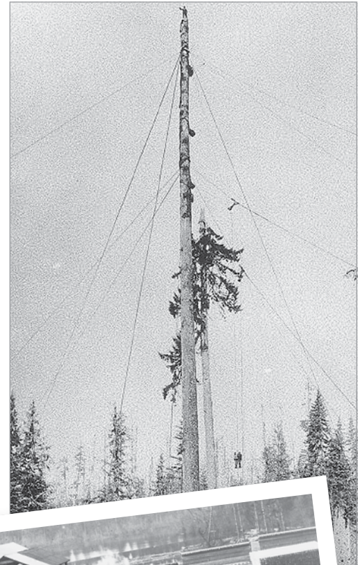
Left: Employment at the Lake Sawyer Lumber Company ranged from 20 to 30 men producing 40 to 50 thousand board feet per day. Above: The Lake Sawyer Mill Company log dump, circa 1928, at the southwest end of Lake Sawyer where the Sunrise Resort is today. Right: This photo was taken in 1926 of a logging spar used by the Lake Sawyer Mill Company. Note the man standing on top and the two men dangling from one of the cables. Bottom right: Stacked lumber at the sawmill.
