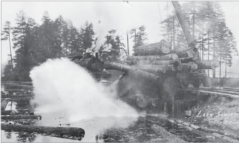
Left: Employment at the Lake Sawyer Lumber Company ranged from 20 to 30 men producing 40 to 50 thousand board feet per day. Above: The Lake Sawyer Mill Company log dump, circa 1928, at the southwest end of Lake Sawyer where the Sunrise Resort is today. Right: This photo was taken in 1926 of a logging spar used by the Lake Sawyer Mill Company. Note the man standing on top and the two men dangling from one of the cables. Bottom right: Stacked lumber at the sawmill.
