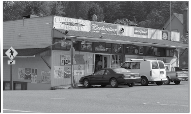
The Cumberland Grocery is little changed almost 95 years later except that the post office that was once inside is now long gone. (Photo: Robert Dobson)
