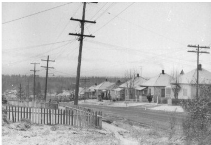
Houses from the Lawson Mine were moved to current-day Lawson Street, here shown circa 1950.
