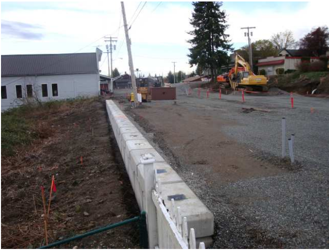
Retaining wall between the Book Store and the Smoke House
