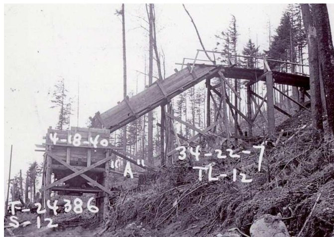
Elk Coal mine workings April 1940 – from the King County Assessor archives
