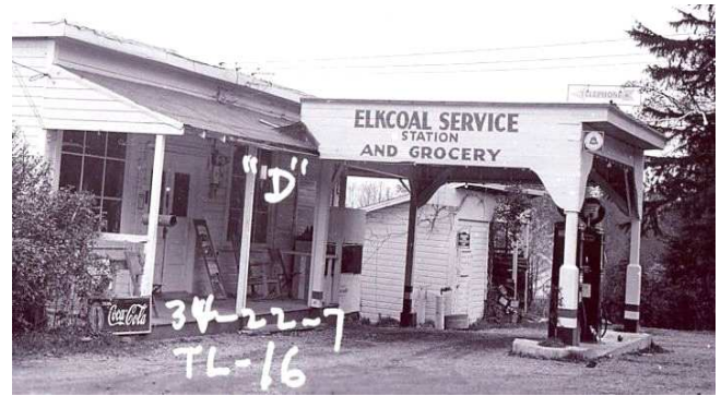
Elk Coal Service Station and Store April 1940 – from King County Assessor archives
