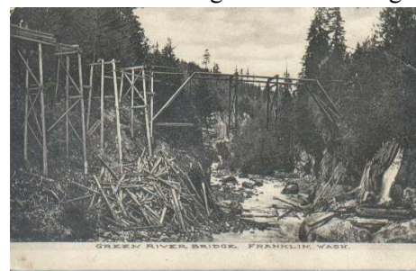
Pre-1900 Franklin-Green River original wooden truss Bridge under construction. Courtesy of the Black Diamond Historical Society.
