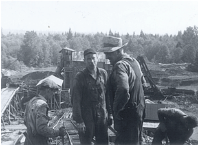
Mine #11, Aug 1949, rock dump work. L to R: Harold Lloyd, Archie Eltz, Frank Merritt, Carl Falk. (Photo courtesy of Bill Kombol)
